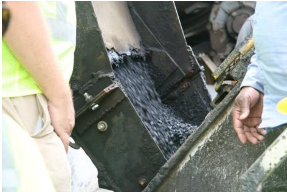
Drum Exit / Slat Conveyor
